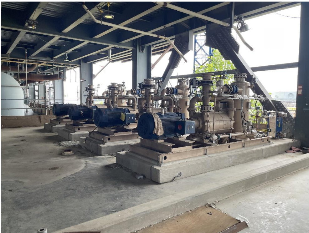
Turbine Building installation
