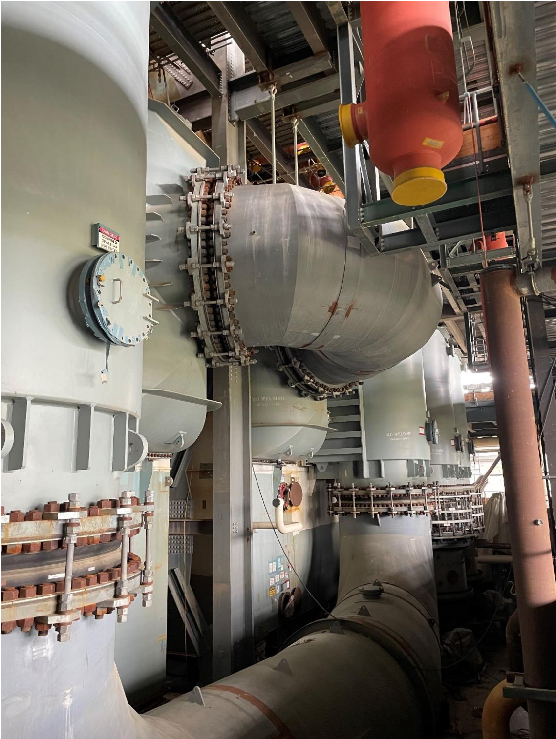
Turbine Building installation
