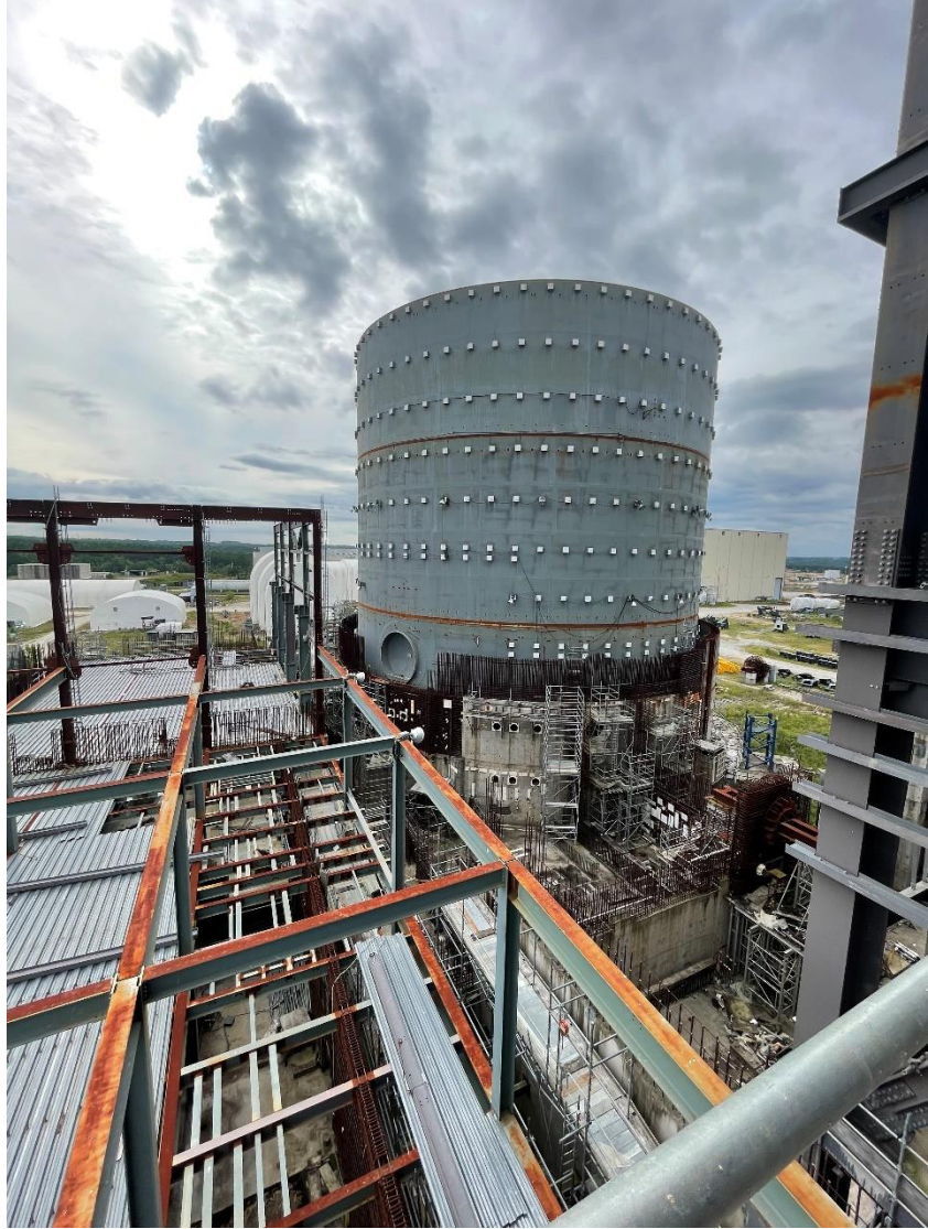
Additional view of Reactor 2 containment structure
