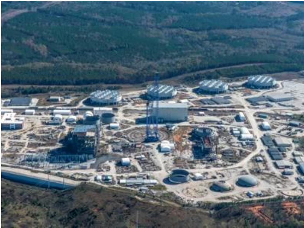
Site Overview (Unit 2 Left, Unit 3 Right)
