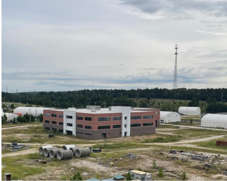
Administration Building (Completed) awaiting sewer system hook up
