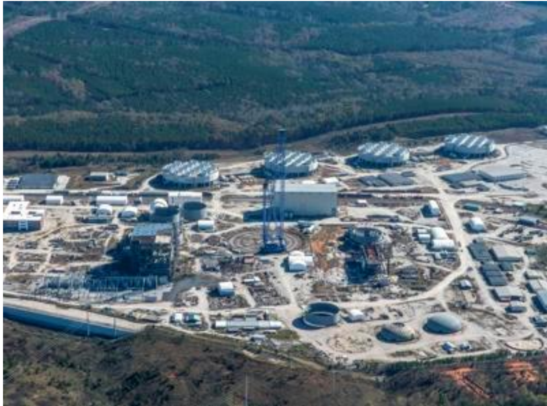
Aerial view of the inactive V.C. Summer Nuclear Plant Site
